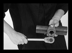
Hold the coupling in position and tighten the nuts alterna-tely and equally leaving equal gaps between the U-bolt pads. Apply specified torque to ensure proper sealing.
