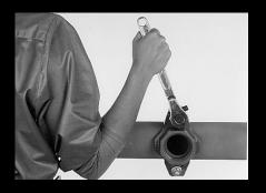
Tighten the nuts alternately and equally leaving equal gaps between the bolt pads. Apply specified torque to ensure proper sealing.
